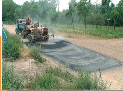
*The method enables to obtain strong, weatherproof ground beds and road coating without using the expensive imported rock materials due to the local soil property regulation*
