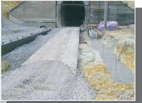
*The purpose: The smooth changes of rigidity under the metal ground bed at its jump up to 6-8 times in the zone of joining the unballasted permanent track with the conventional one on the ballasting.*
